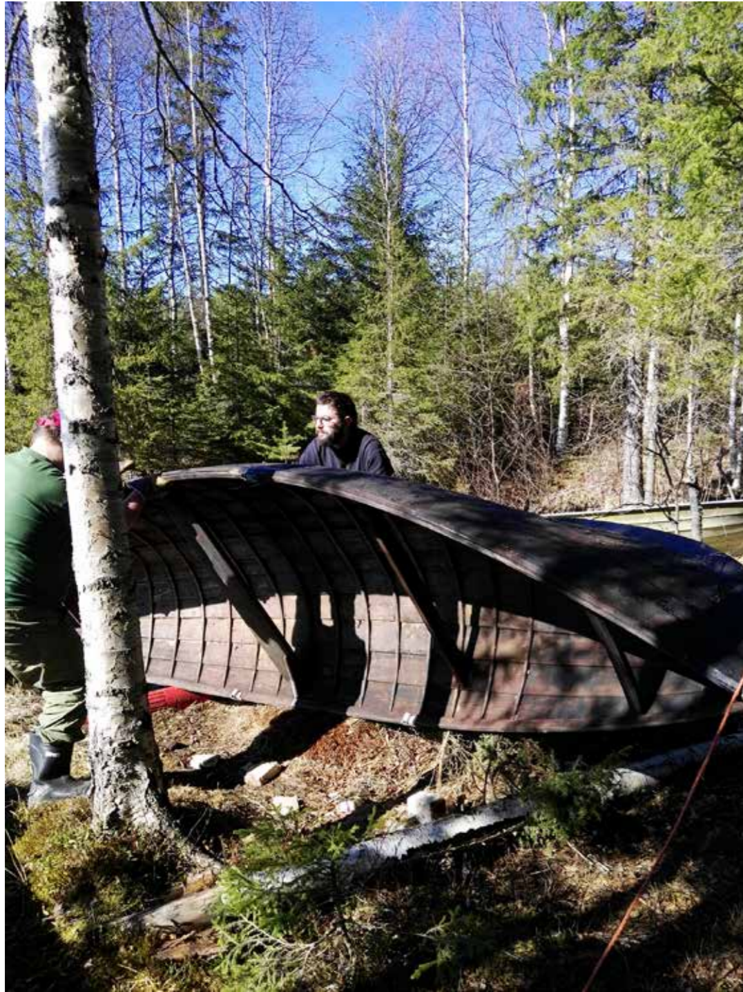
Seining boat restoration with traditional methods (turvottaminen) using pine tar (terva). Image courtesy of the artist.
